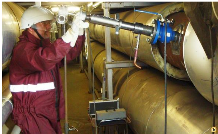
drilling procedure certified for district heating applications (“hot tapping”)
