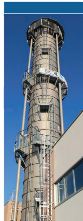
Stainless steel piezometric tower for the calibration of large DNs
